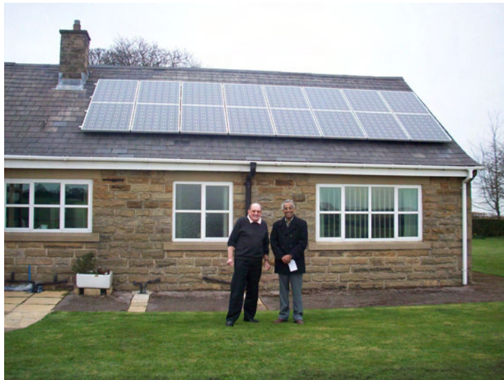
Proud owner of the solar roof, Frank Gilliver facing the camera with Professor Dharmadasa.
