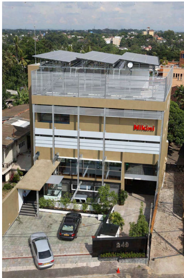
The Nikini building powered by a solar roof connected to the National Grid
