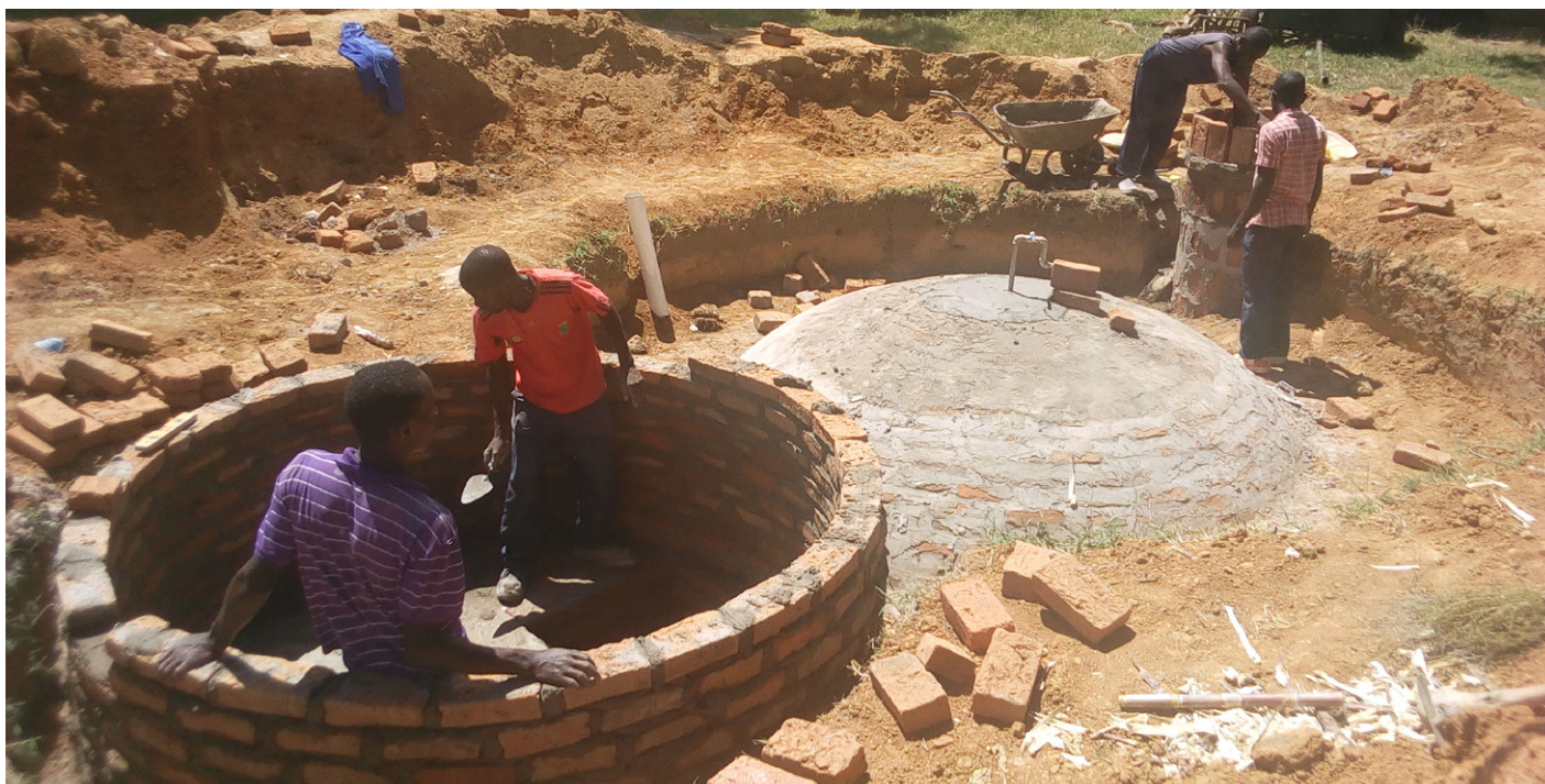
Biodigester construction at Chadiza Boarding Secondary School.
