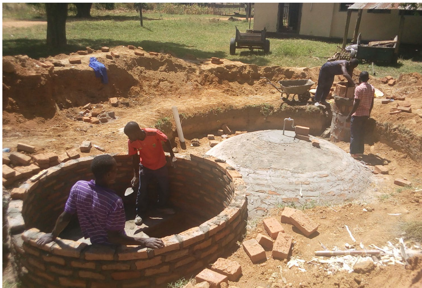
Biodigester construction at Chadiza Boarding Secondary School.
