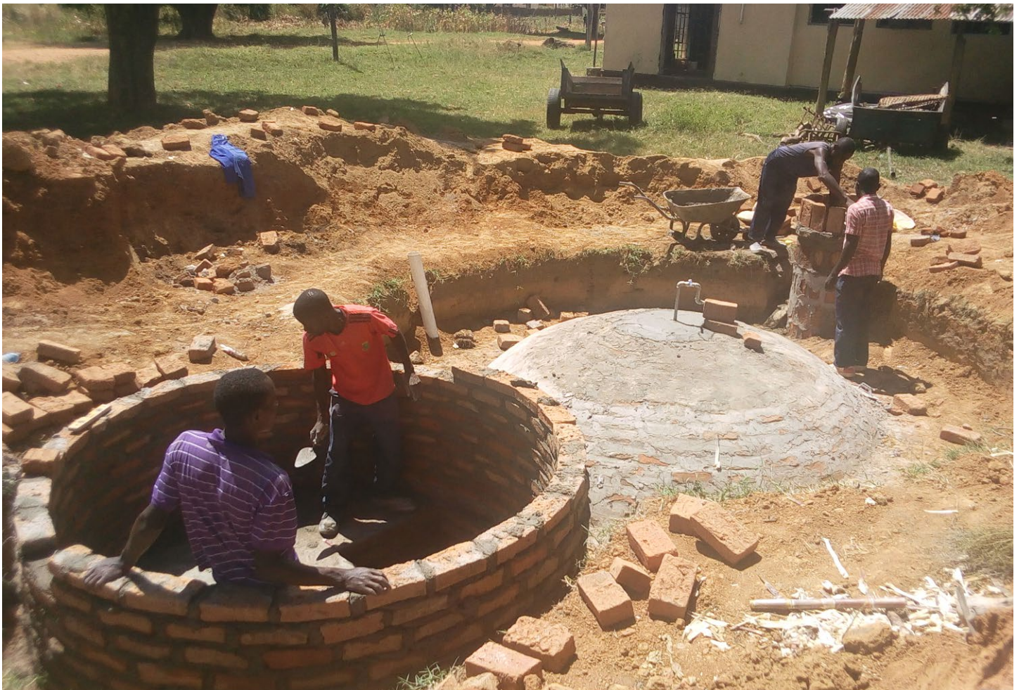
Biogas digester construction at Chadiza Boarding Secondary School.
